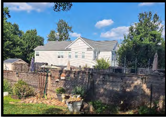
View of the West Side Plane of the Roof
