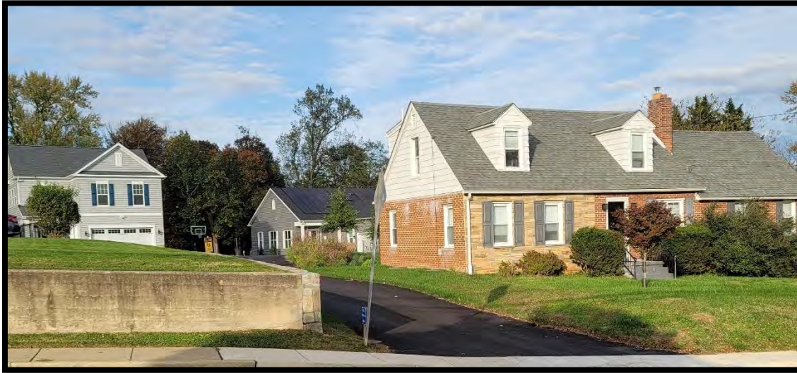
The Hebron House Historic District Looking North from Martins Lane - View of Historic Hebron House in Front, 21 Martins Lane (Left) and 19 Martins Lane (Right) in the Rear.
