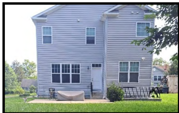
View of the Rear of the House (Roof not visible)
