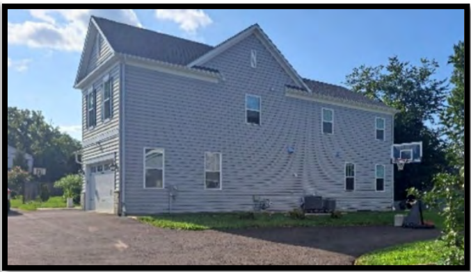
View of the East Side Plane of the Roof
