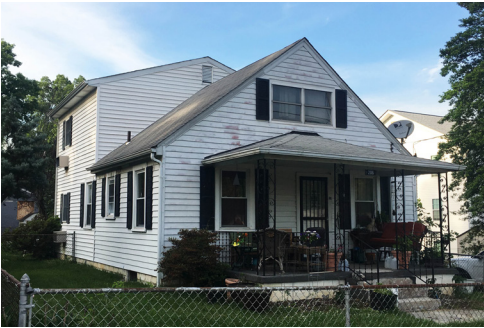
Set-back addition which does not dwarf original house and a roof ridge that is only a few feet above the existing roof is inconspicuous from the street.
