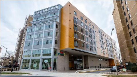
Main Street Apartments 70 units ( Built 2020 )
