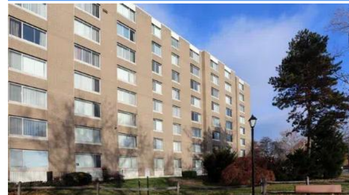
Project: Bethany House (Preservation)
