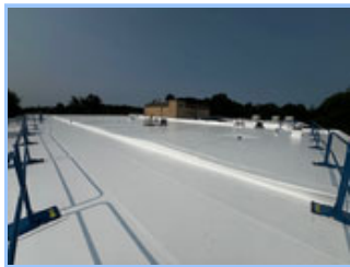
Newly replaced City Hall roof
