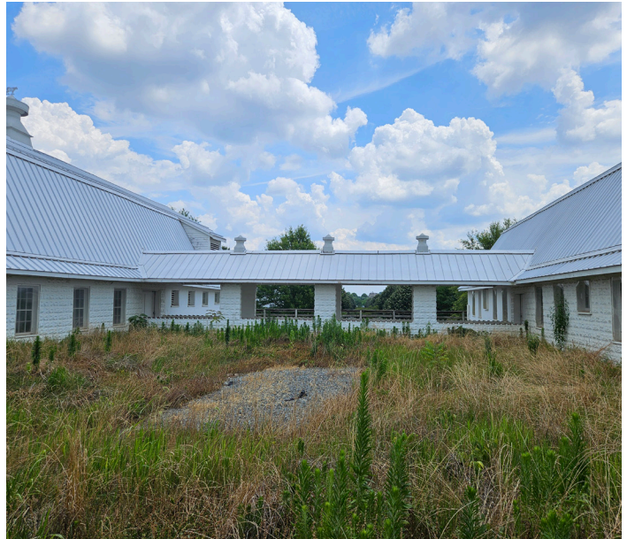
Existing courtyard looking east
