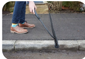
Model 3: Resident Installed Charging Duct/ Cord
