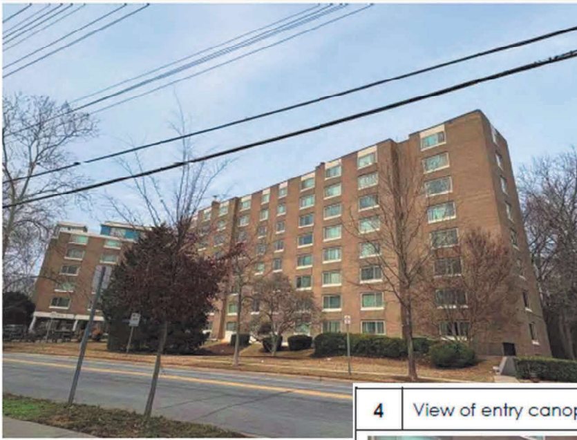
1 View of Building from Rollins Avenue.
