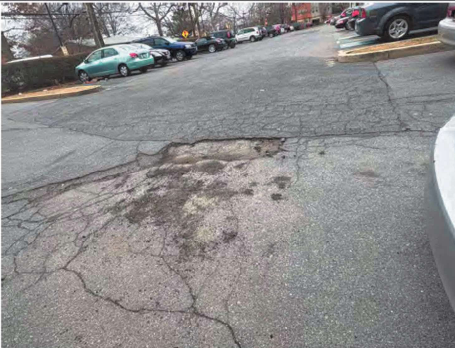
16 Cracks observed in asphalt sections throughout.
