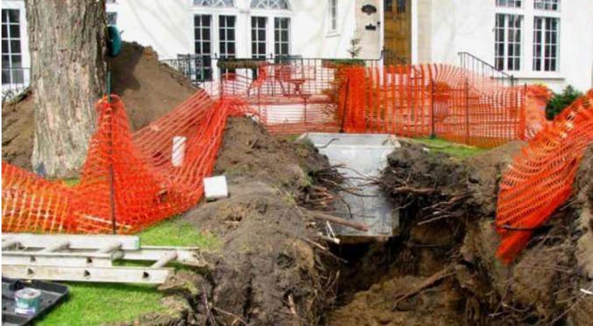
Figure 25: Note that the face of excavation is typically ragged and the roots to be pruned are at varying setbacks. Pruning only required on left side (one payment line) where the live roots exist.
