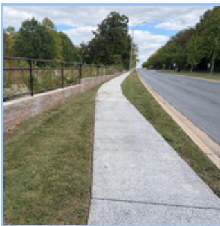
Recent sidewalk construction on W. Gude Drive
