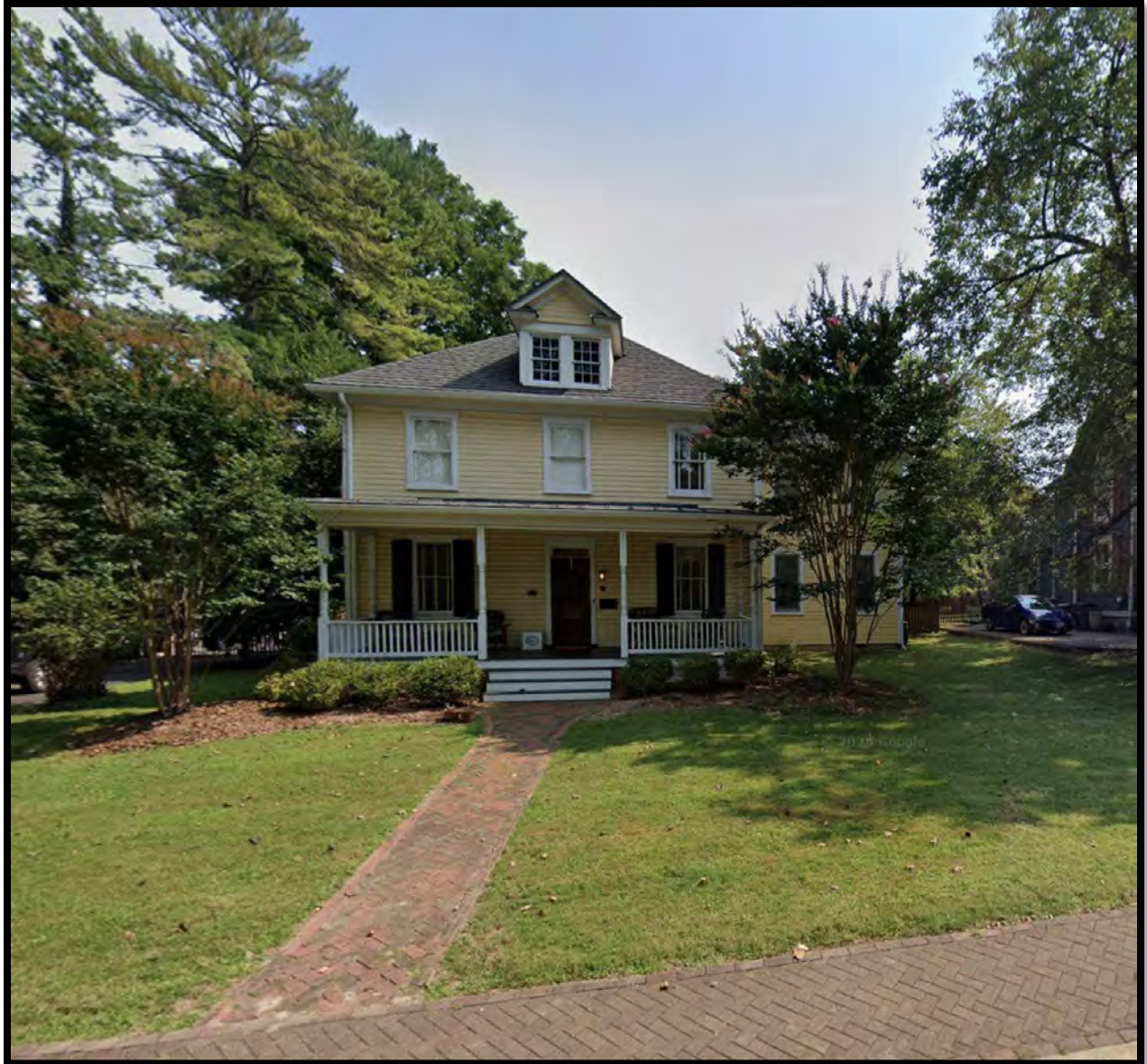
Figure 2: Front Facade (West Elevation), showing front porch steps to be replaced, along with addition of handrails.
