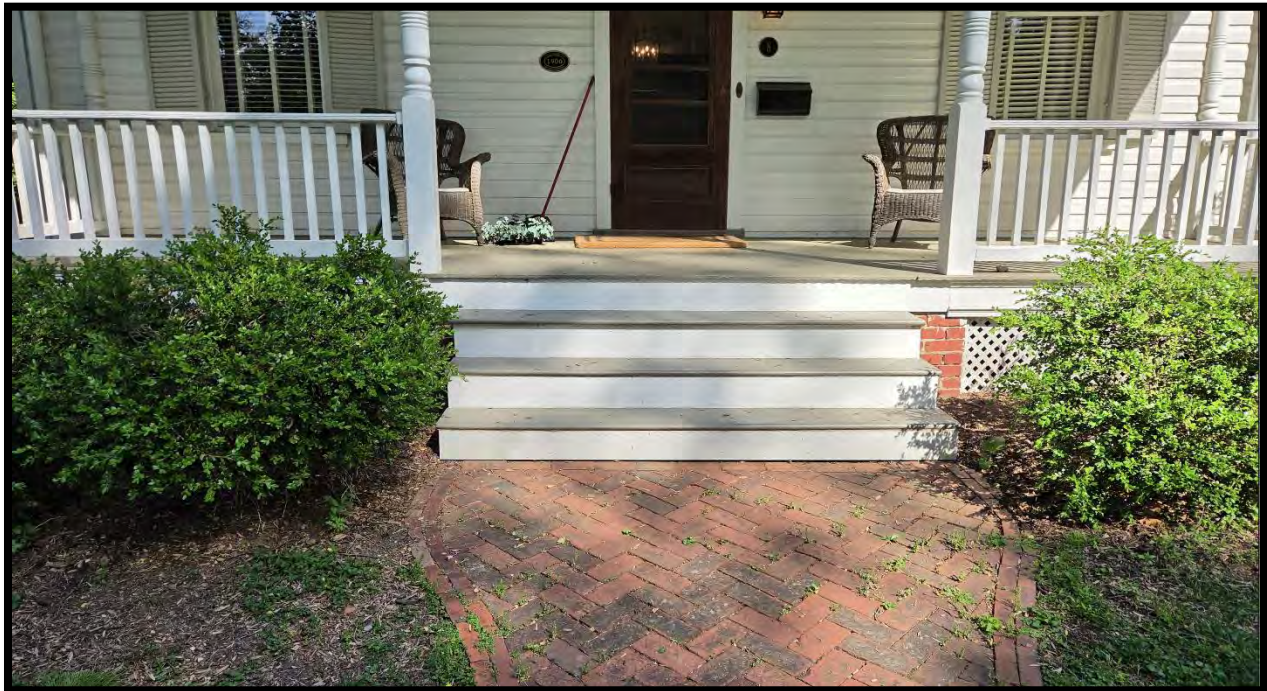
Figure 3: Existing Condition of Front Steps (West Elevation)
