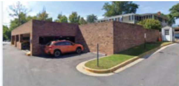
4. Garage West Elevation View from the parking lot looking West
