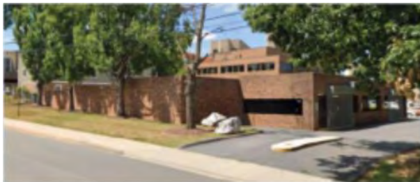
3. Garage View from Fleet St Facing the 1953 parking garage structure
