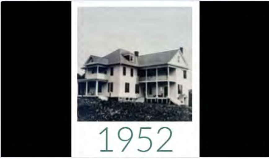
Hege House (1952) Original state prior to modernization.
