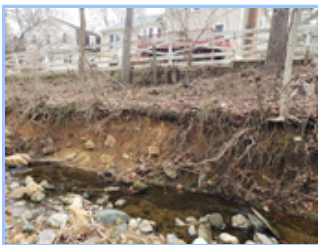
Stream bank erosion along Glenora Park Stream
