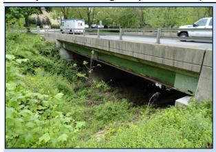
**Description:** This project plans, designs, and constructs the replacement of the Hurley Avenue bridge near the Watts Branch Parkway intersection. This bridge was constructed in 1969 and requires replacement. The planned improvements will increase the structure's longevity and live load carrying capacity.
