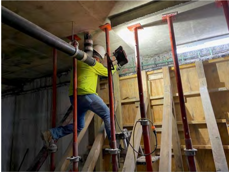
Photo 3: DPR Placing Concrete at Approved Repair Patch
