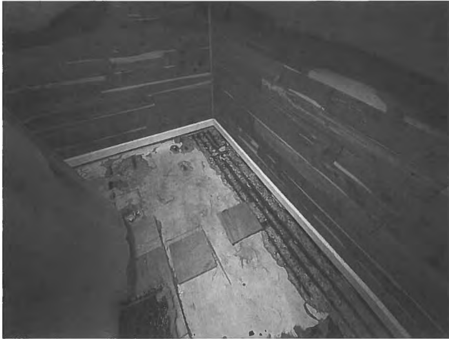
Photo 2 – SK&A Observing the Interior Walls of the WIC During Water Test. No Leaks were Noted
