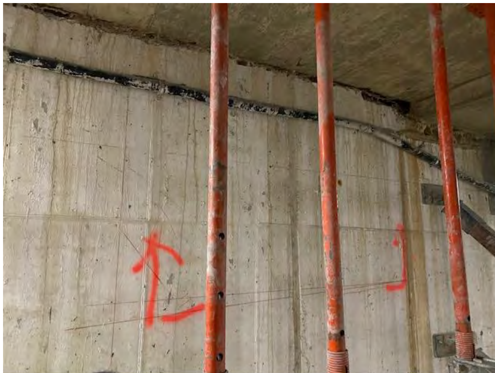
Photo 2: Overview of Vertical Foundation Wall Repair #2
