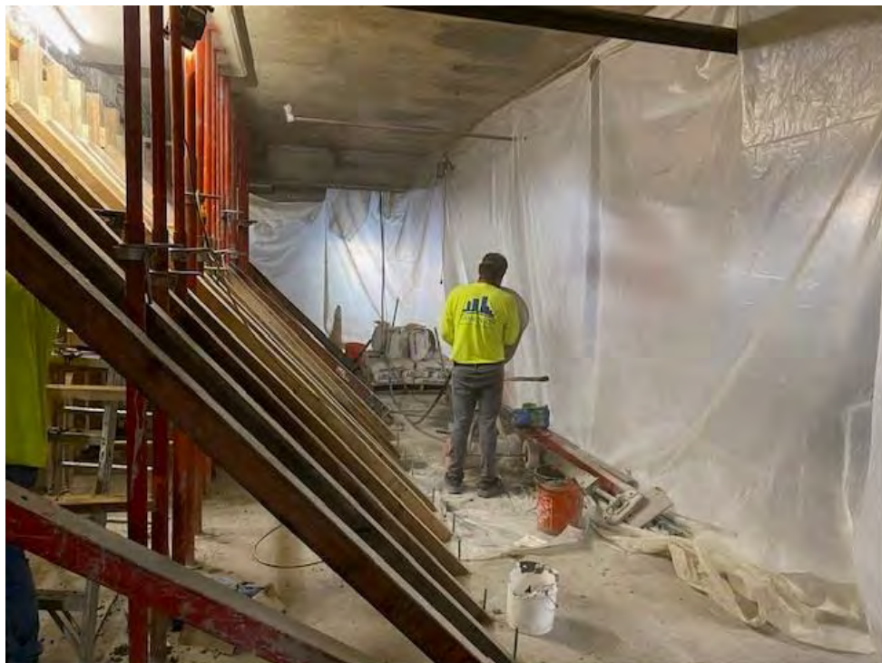
Photo 2: DPR Batching USCP Deck Mix AE
