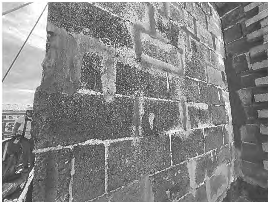
Photo 2 – View of Parged CMU Back-Up Wall West Elevation
