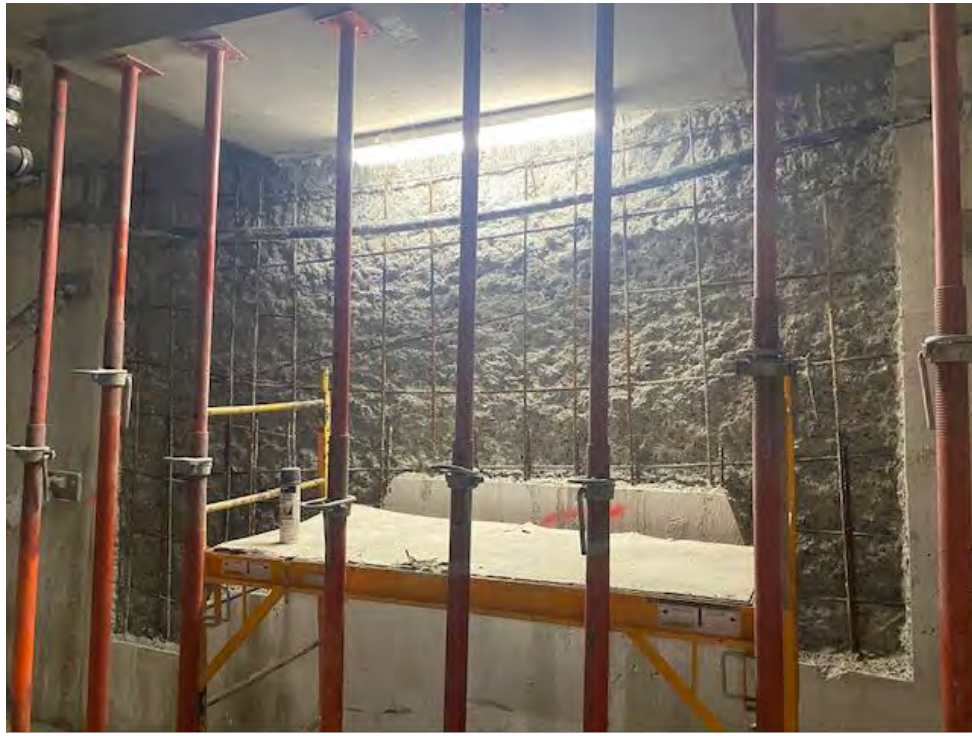
Photo 1: Overview of Vertical Foundation Wall Repair
