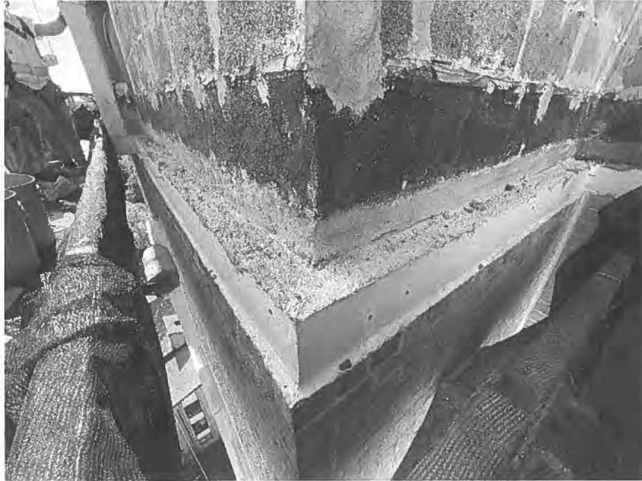
Photo 3 – View of Removed Existing Through-Wall Flashing at Top of Slab and Back-Up Wall Interface
