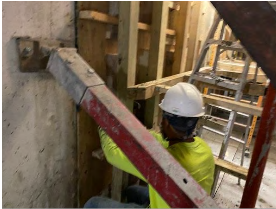
Photo 4: DPR Consolidating Placed Concrete with Hammer
