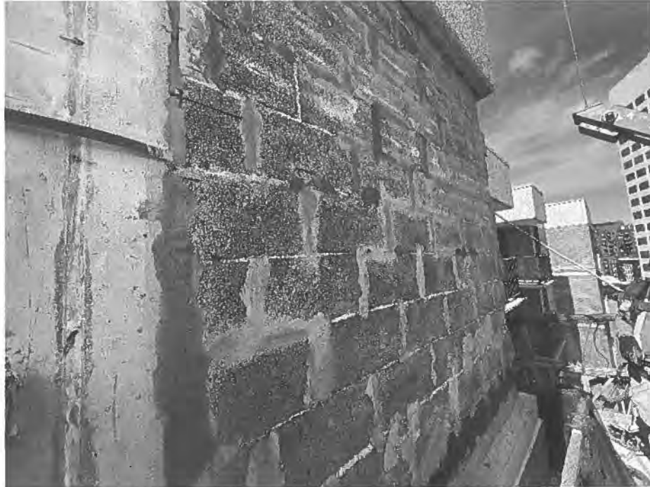
Photo #1 – View of Parged CMU Back-Up Wall North Elevation
