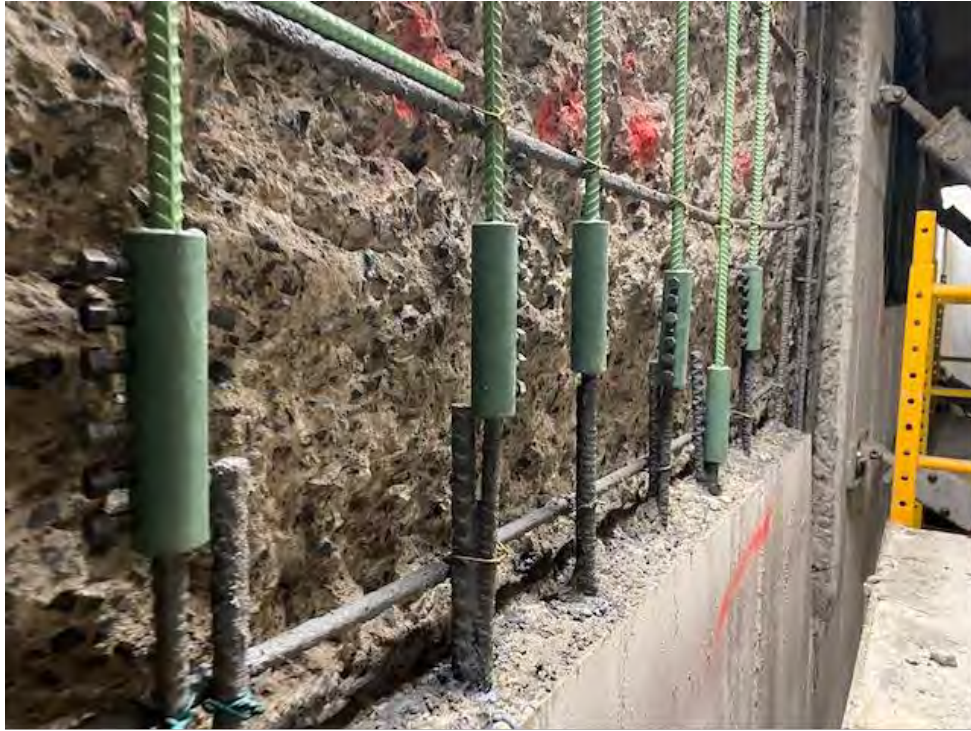
Photo 2: Approved Reinforcing Coupler Being Used at Vertical Foundation Wall Repairs
