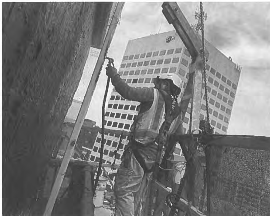
Photo 1 – EVAT Applying Water to the North Wall of the Unit 4-1302 WIC
