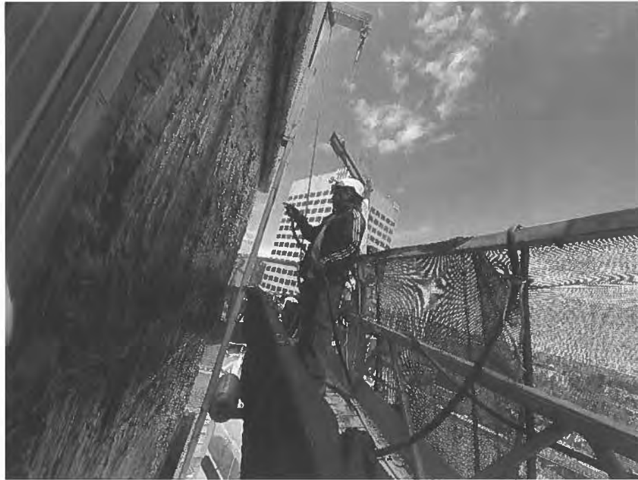
Photo 4 – EVAT Applying Water onto the Waterproofed Backup Wall
