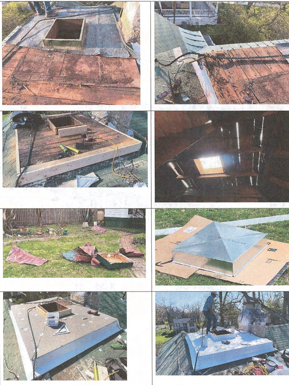
Figure 4 to Figure 11. Work in progress photos.
