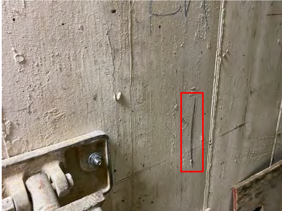
Photo 3: Location Marked Within Red Where SK&A Instructed DPR to Capture within Bracing
