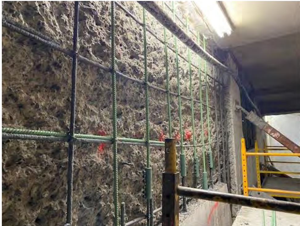
Photo 1: Overview of Marked Reinforcement Replaced Per Project Details
