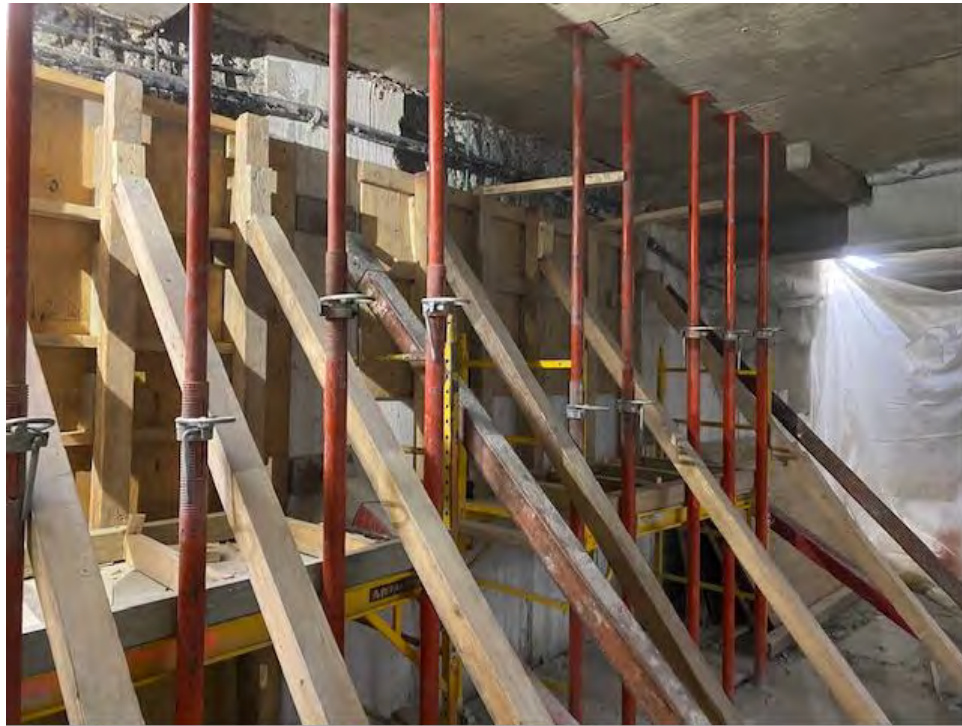
Photo 1: Typical Formwork Installed at Foundation Wall Repair Patches
