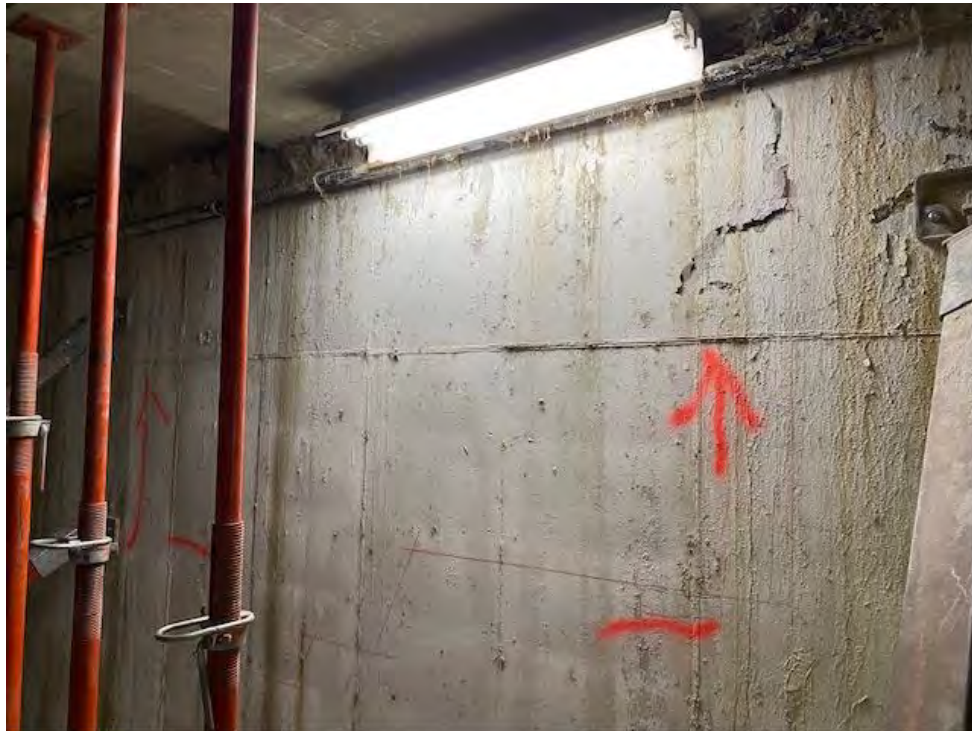
Photo 1: Overview of Vertical Foundation Wall Repair #1
