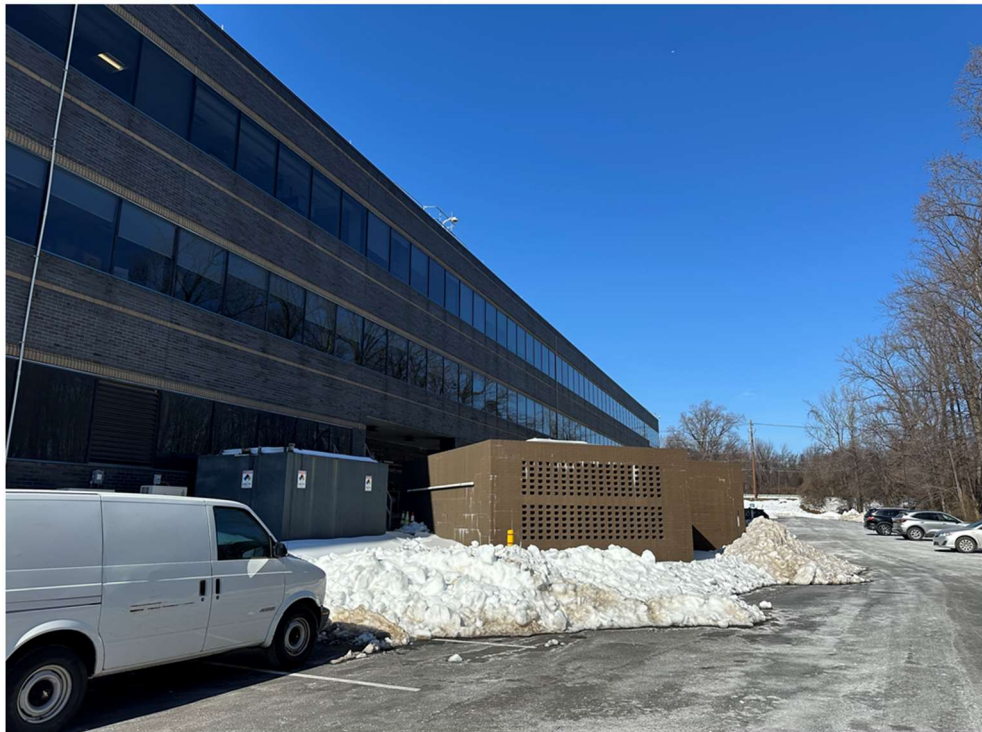
Figure 6 - 1 Curie Court, Rear/North Elevation
