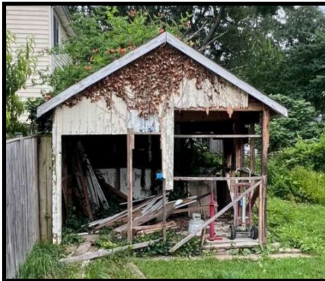
Former Shed Front
