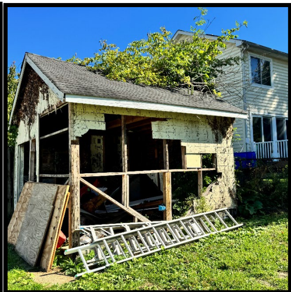
Former Shed Side
