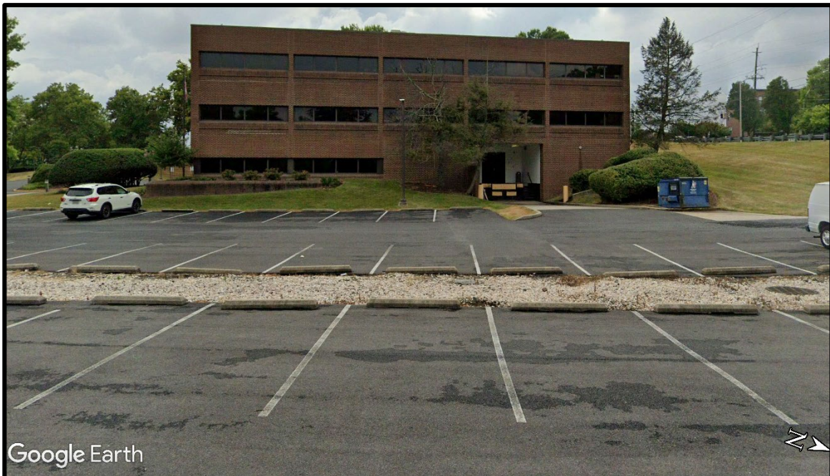
East Side Elevation from Parking Lot
