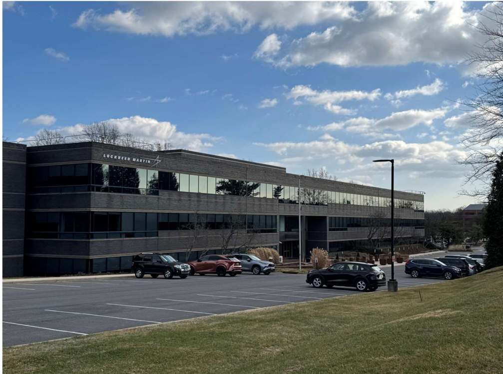
Figure 4 - 1 Curie Court, Front/South Elevation
