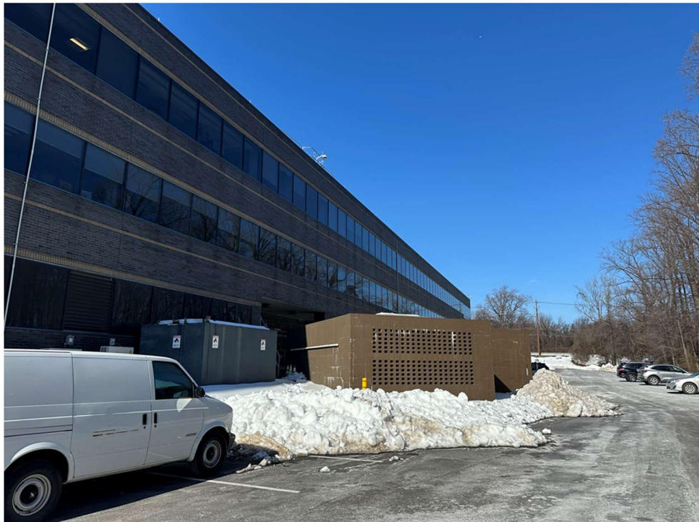
Figure 6 - 1 Curie Court, Rear/North Elevation
