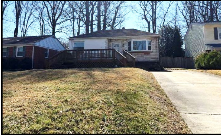
Front (southwest) elevation.
