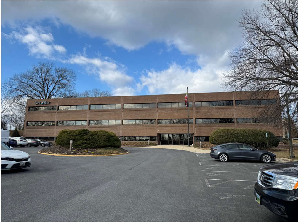
Figure 1 - 1395 Piccard Drive, Front/East Elevation
