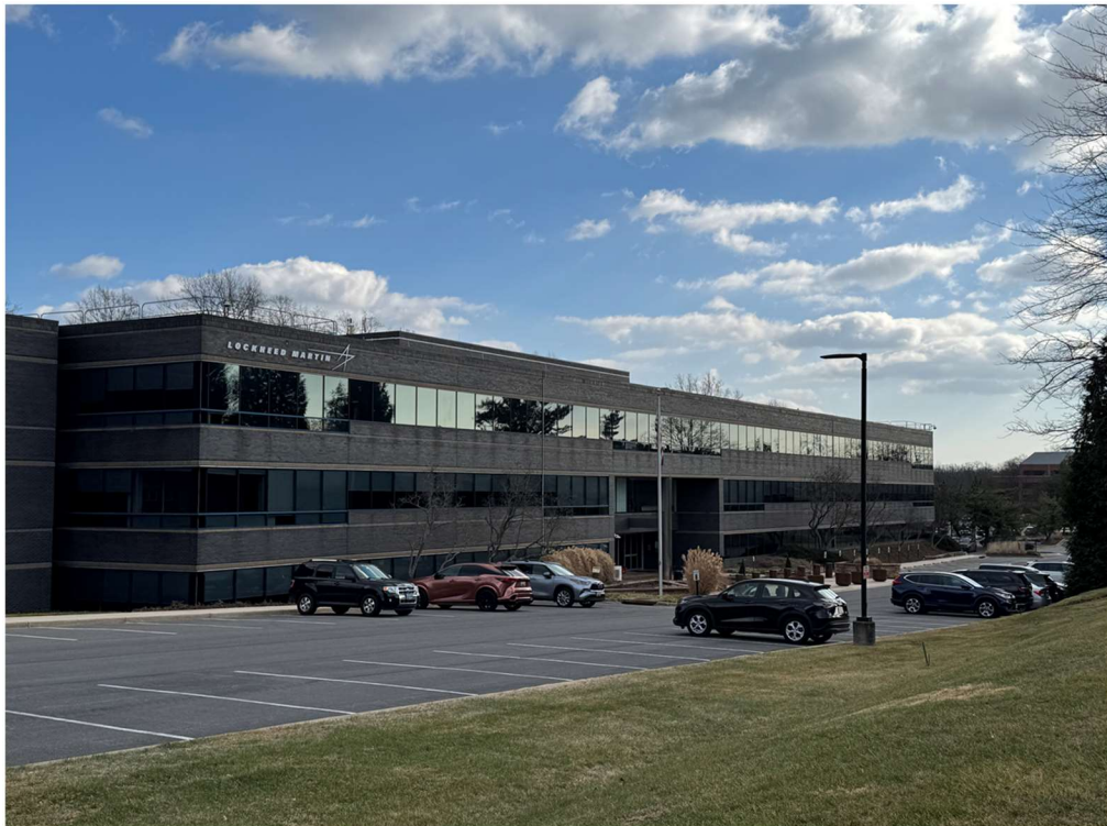
Figure 4 - 1 Curie Court, Front/South Elevation
