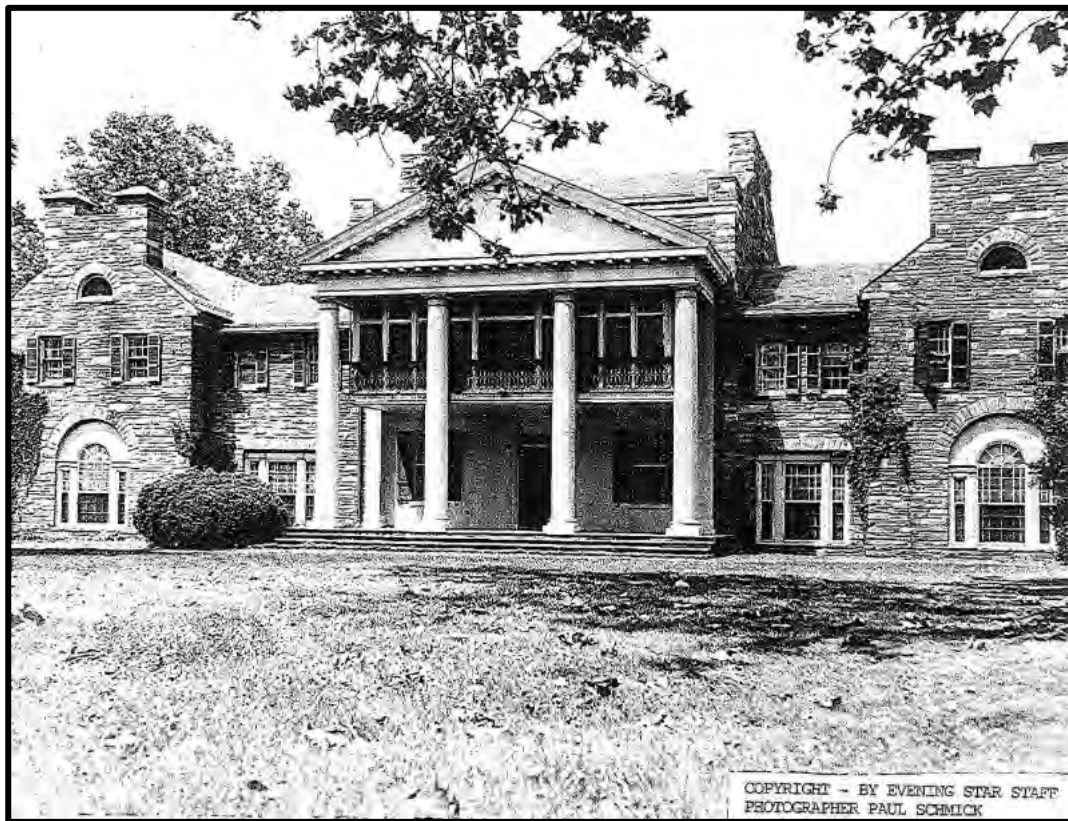
Figure 5: 1926 View of Glenview Mansion, South Elevation
