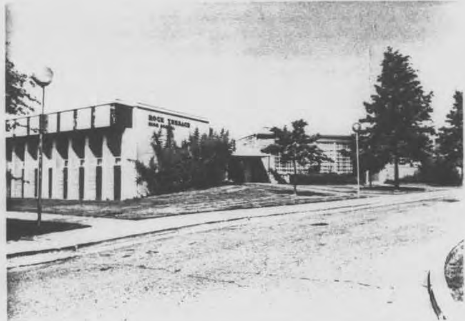
ROCK TERRACE SCHOOL 390 MARTIN'S LANE
