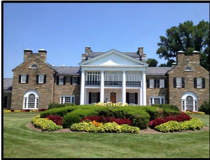
Figure 4: Older View of Boxwoods (c. 2015), South Elevation
