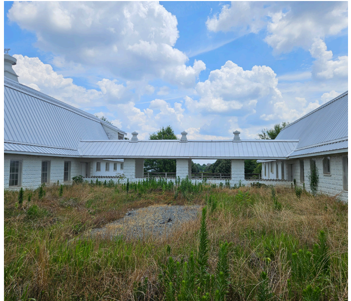
Existing courtyard looking east
