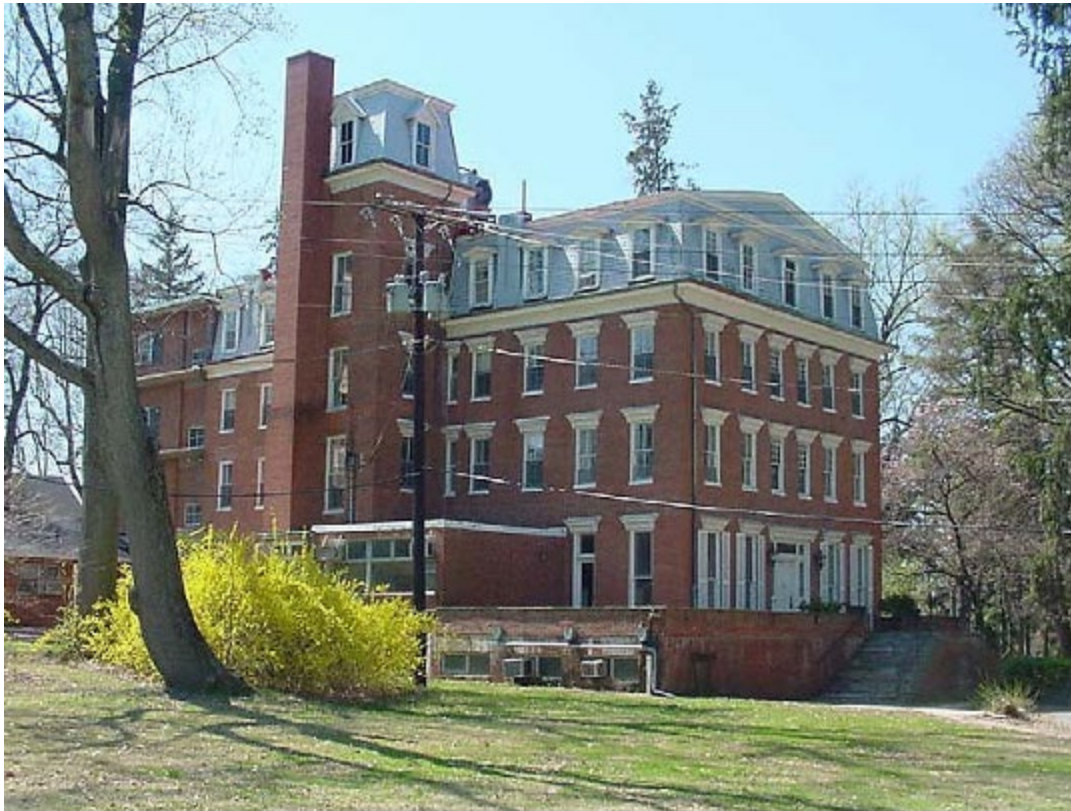
North and East Façade Woodlawn Hotel/Chestnut Lodge - 2003
